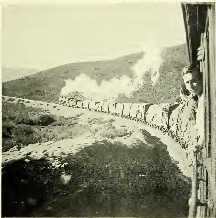
RAILWAY TRANSPORT OF PORTLAND HOSPITAL OVER HEX RIVER PASS.
